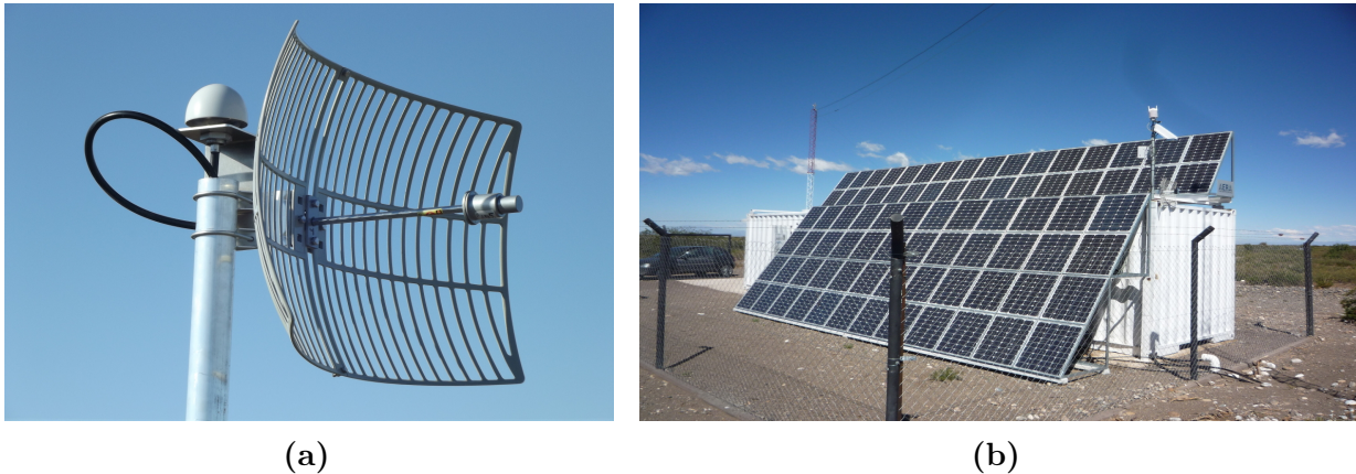
Figure 6.5: Pictures of a wireless communication antenna and a GPS receiver as used for phase II (a) and the CRS container with solar panels (b). The pole with the weather station, the electric field mill and the lightning protection tower are visible as well.
